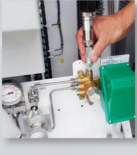
Regardless of the breaker type, installing an SF6 sensor is easy. Sensors can be installed directly into the pipe feeding a pressure gauge, into the breaker's SF6 fill port using INCON<sup>®</sup> Fill Port Adapters, or into a breaker's accessory port.
